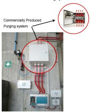
Figure 8 – Commercial purging system
